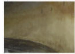
**Fig 6:** After the program, white-water chest walls are clean with no deposition
