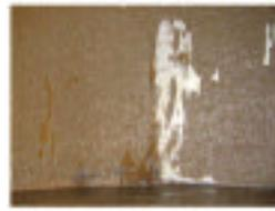
**Fig 5:** Before the program: walls of white-water chest show high levels of deposition
