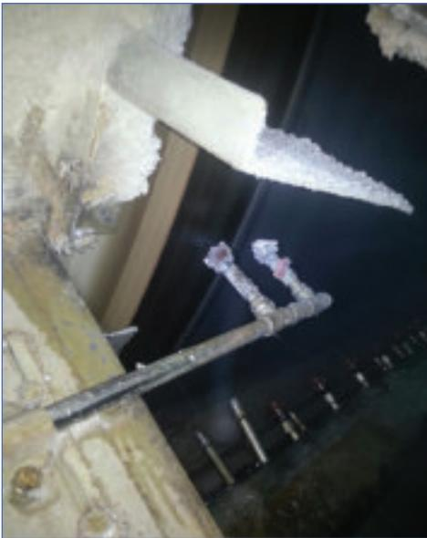
Figure 3: Typical adjustable edge spray in use
