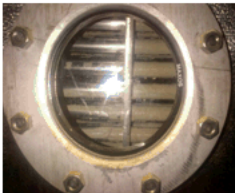
Nine Days After Running Without Infinity SL4393 Scale Inhibitor.
